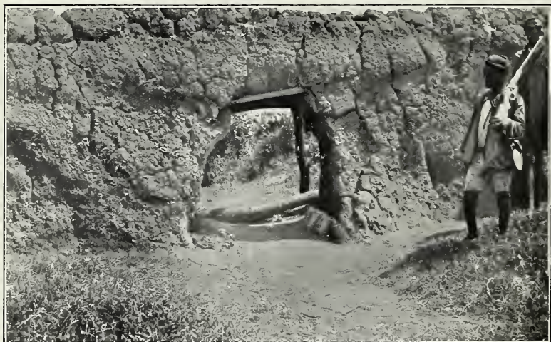
FORTIFICATION OF KISHI VILLAGE (SHOWING ENTRANCE GATE).
